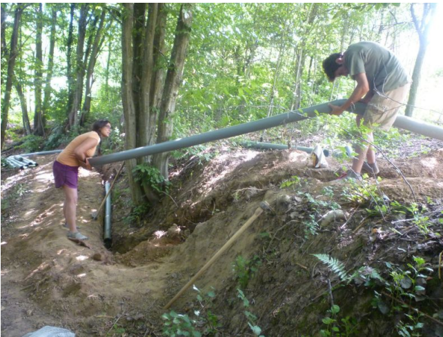
Pipes for rain and shower water into the forest
